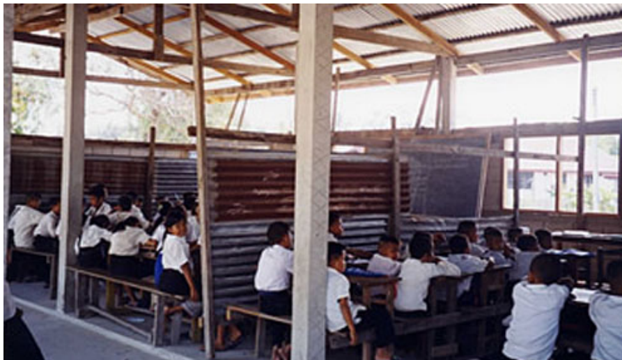
Image 6: Former classroom "walls"
