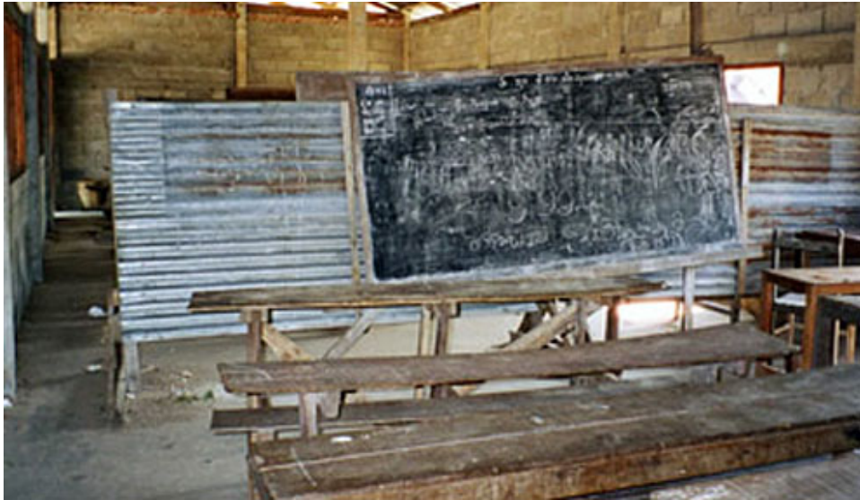
Image 5: The former classrooms
