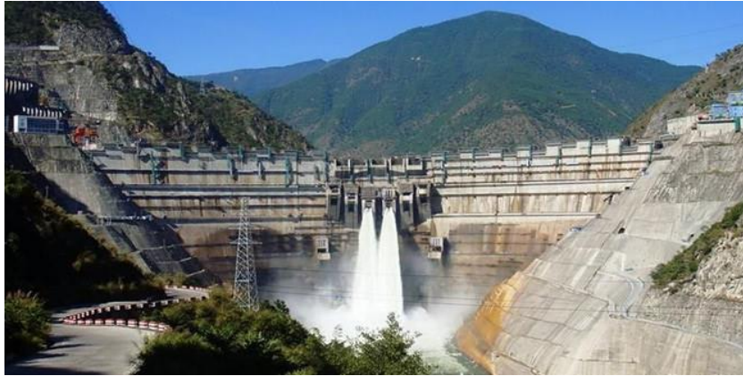
Fig. 5: Hydroelectric power station in Laos (J&C Services)
